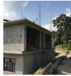
RCC Frame structure with block infill walls
