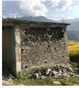
RCC Frame structure with stone infill walls
