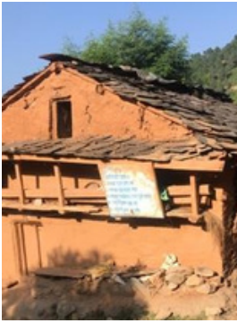
Stone in mud with pitched roof with slate stone
