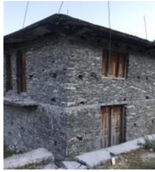
Stone Masonry with RC Rigid Floor (local word for “Linter”)
