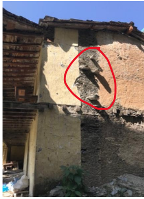
Corner stones are placed in traditional construction technology
